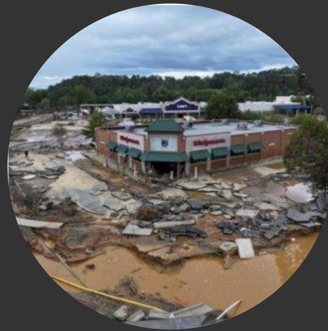
Hurricane Helene Flooding Damage, 2024
